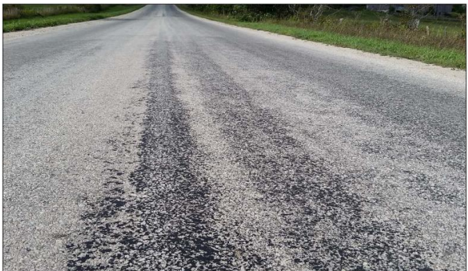
Flushing of pavement
