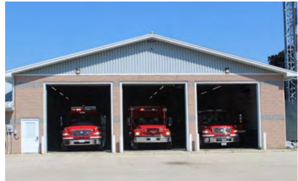
Figure 20: Chelsey and Area Fire Station
