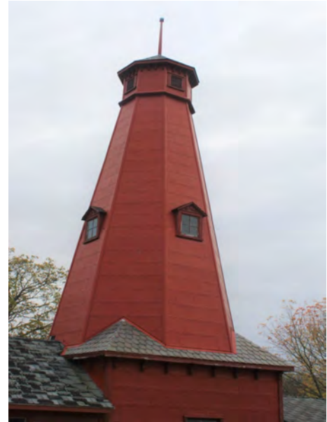
Figure 6: Historic Hose Tower in Paisley
