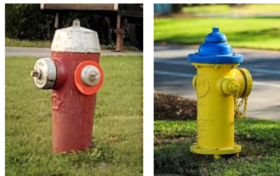
Figure 12: Colour-Coding of Hydrants
