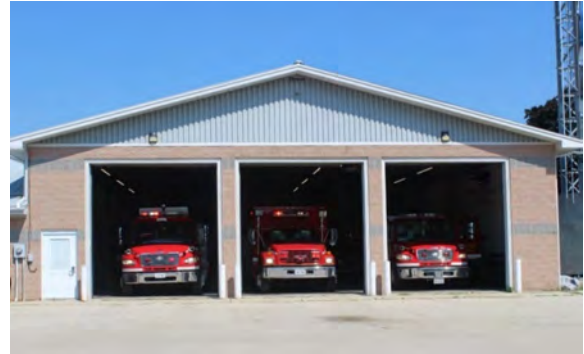
Figure 20: Chelsey and Area Fire Station
