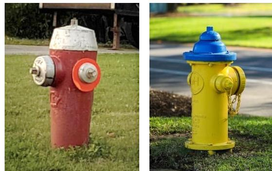
Figure 12: Colour-Coding of Hydrants
